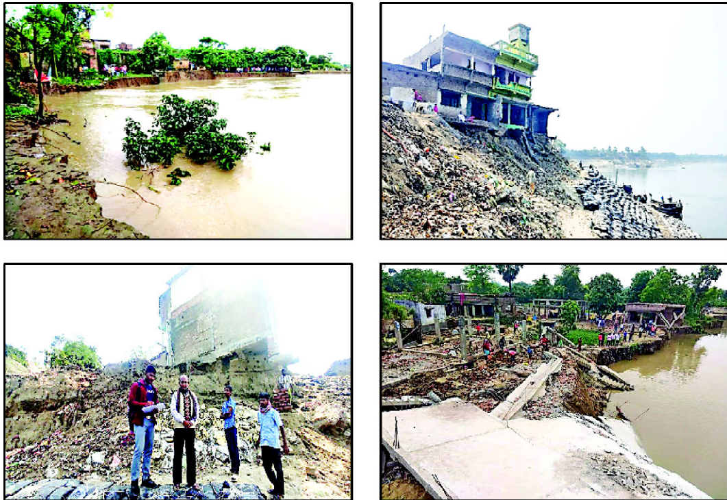
Fig. 2: Severity of the bank erosion problem in Dhusuripara Census town.
